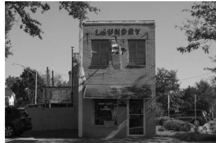
C: GOVERNORS AVENUE, NEIGHBORING BUILDING
